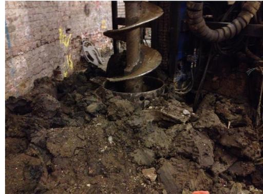
Buildup of spoil leading to uneven ground conditions
