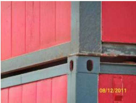
**Photo shows:** View of remaining cabins immediately after incident – cabins are not physically connected or secured to the ground.
